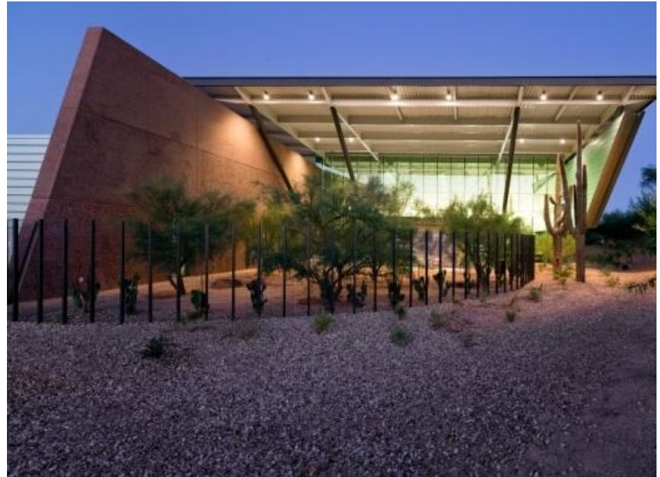
Архитектор: DWL Architects & Planners, Inc. / Douglas Sydnor Architect and Associates Фото: Bill Timmerman
